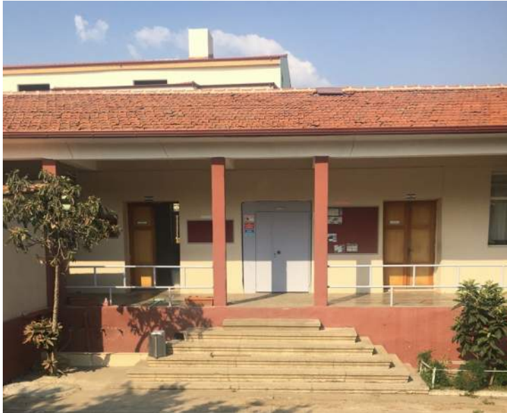
Figure 3.34 Entrance and courtyard of old Ataturk Elementary School (Autor 2017)
