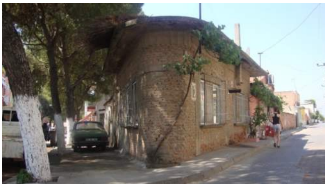
Figure 3.73 One one story and two one story with basement corner houses from Republican Period (Autor 2012)
