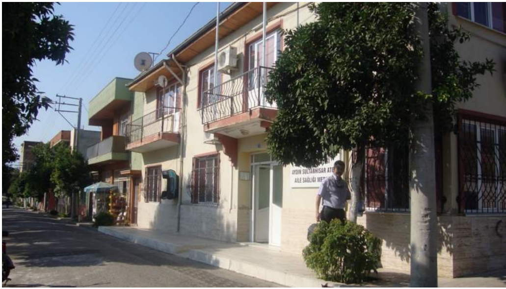
Figure 3.45 Photographs of Sultanhisar Atça Health Center (Autor 2023)
