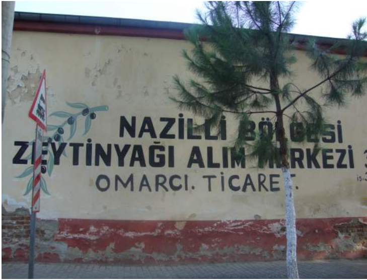
Figure 3.48 Photographs of Nazilli Region Olive Oil Procurement Center (Autor 2012)
