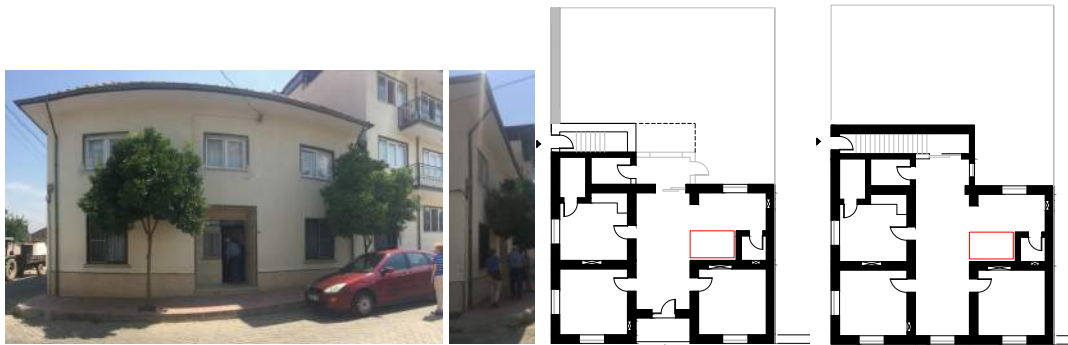
Figure 3.77 Two story Altered Republican Period Building (Autor 2017)
