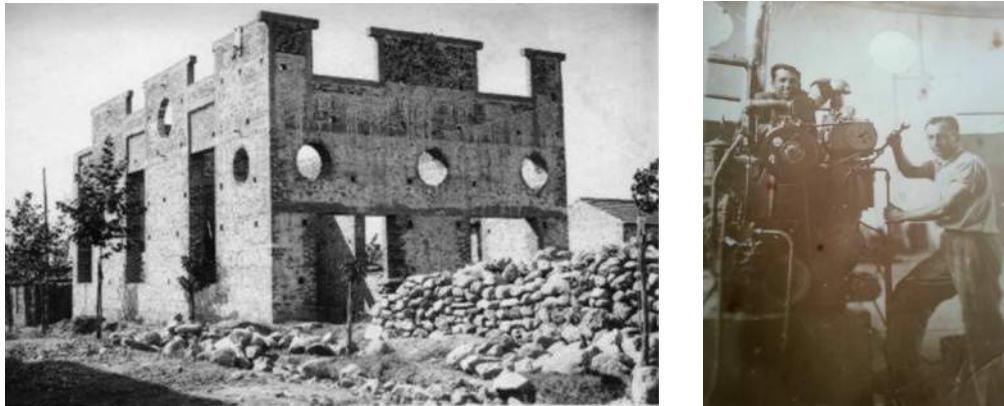
Figure 3.37 Left figure Power Station construction (Atça Municipality Archives) Right figure Inside machinery (Atasoy 2022)
