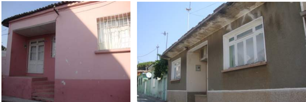
Figure 3.72 One story Republican Period Residential Houses (Autor 2012)
